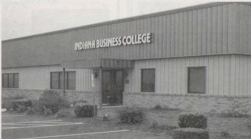
The front of the Indiana Business College building.
