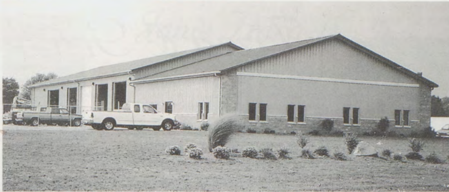
The front of the J.E. Ross Construction building on Raymond Street.
