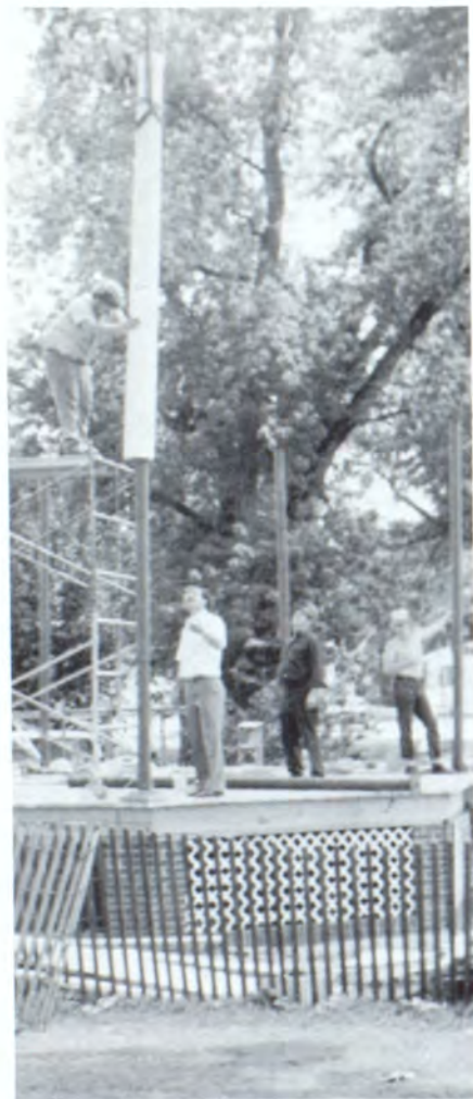
In the process of constructing the bandstand, Mr. Charles Biggs guides the hollow pole that will cover the support beams for the top of the bandstand.
